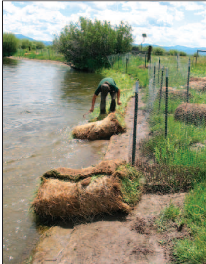
Wetland Sod installation.
